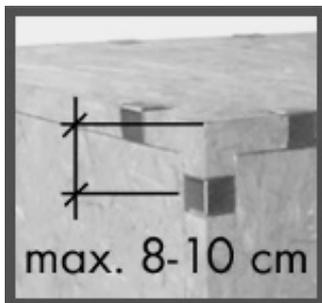
Insert into the groove on one side of the box, press across the corner and hit with a hammer (min.300 g) (slight clicking noise = perfect fit!)
